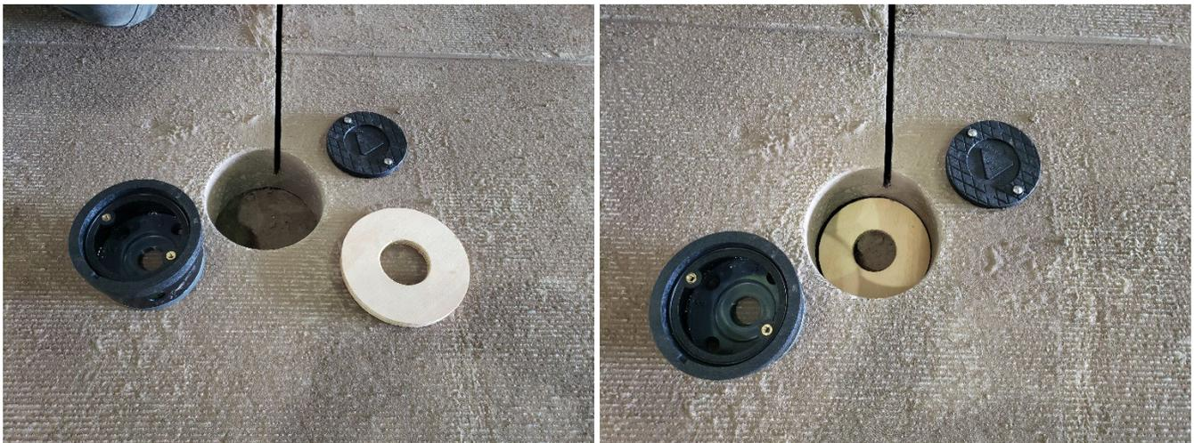
Figure 5: Roadbox and annular piece of wood sitting next to corehole
