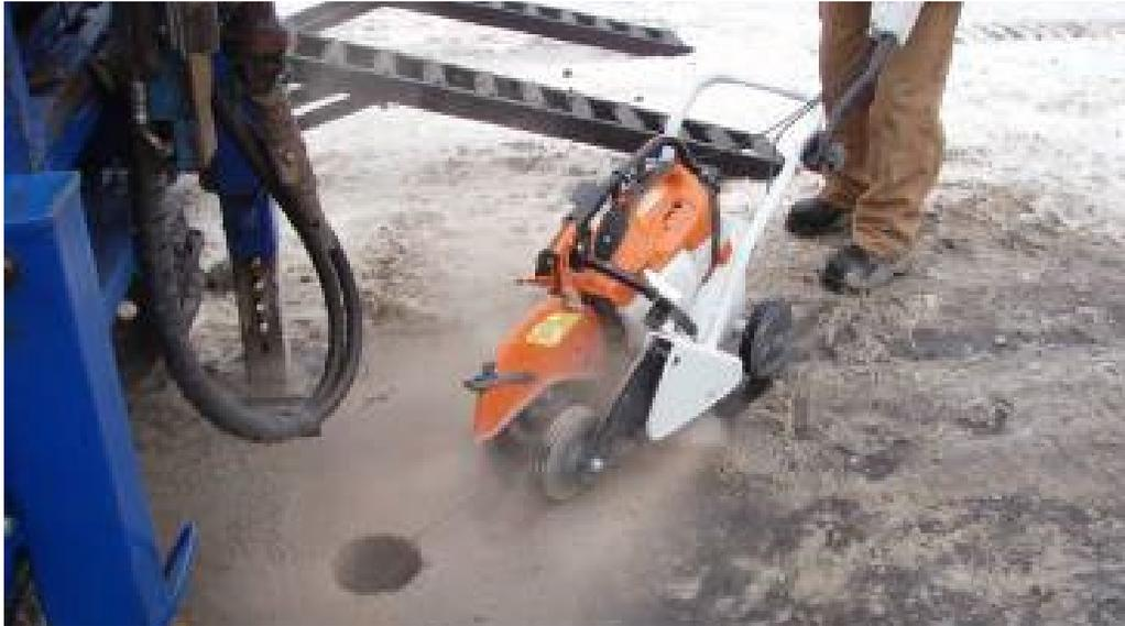
Figure 2: Cutting slit trench into the pavement
