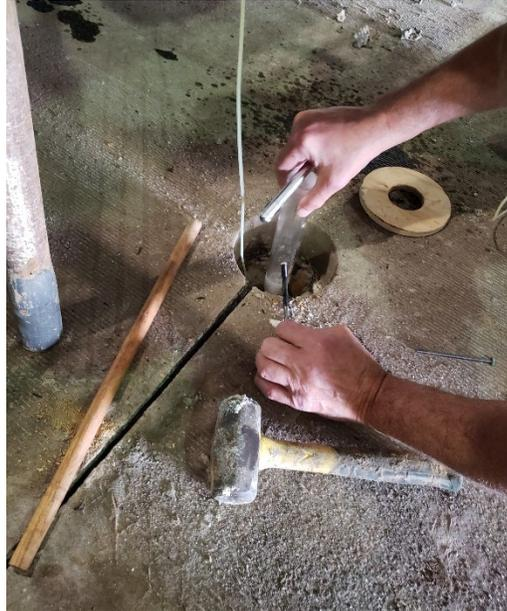
Figure 9: Connecting rod being inserted into the setting tube, in preparation for setting the hydraulic anchor
