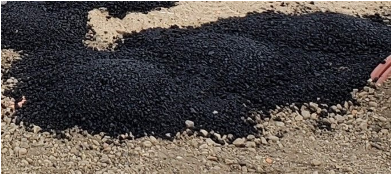
Figure 13: With the top disk reinstalled cover the gage with asphalt again and using your hand pat down the asphalt (as a tamper).
