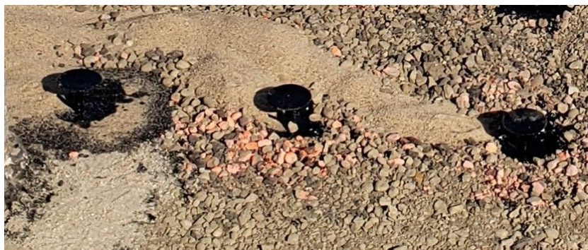
Figure 10: Finish filling sand to protect the sensor cable and near gages.
