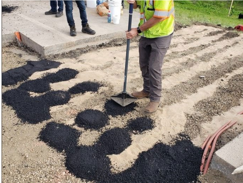
Figure 6: Using a hand tamper, compact or tamp the asphalt and aggregate just enough to tighten up around gage. Caution: Do not tamp too hard.
