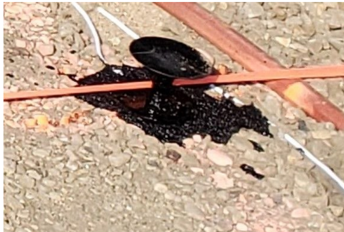
Figure 9: Use mastic to hold gage in a vertical position.
