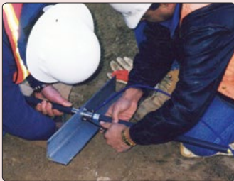
• Attaching the end flange.
