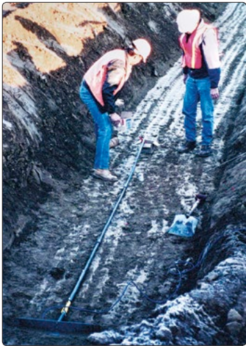
● Installation of Model 4435 sensors.
