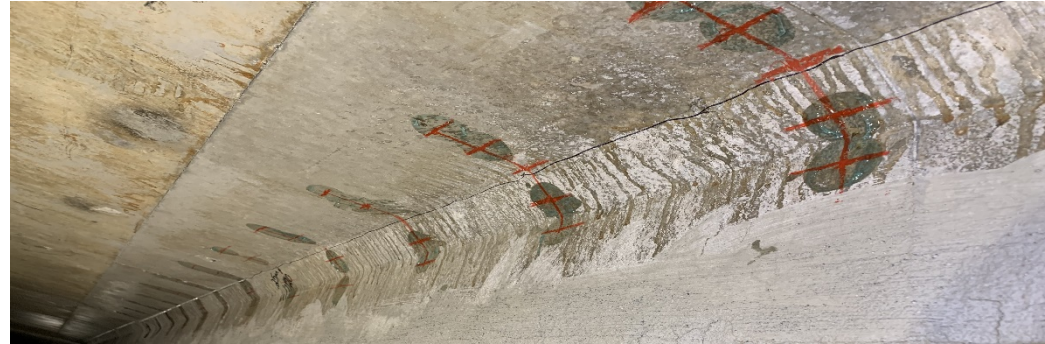
Sample UPV Measurements for Crack Depth
