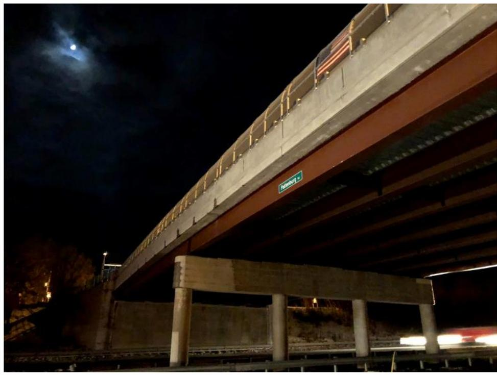
BDI provided load testing services to calibrate an FE model of a newly constructed multi-girder structure. There were perceived large deflections in the multi-girder system and suspected poor construction (designed composite but level of composite action was questioned).
