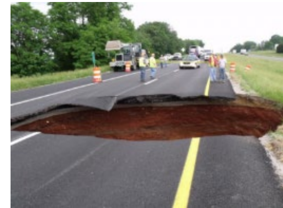
Sinks and their relation to solution cavities beneath the surface.
