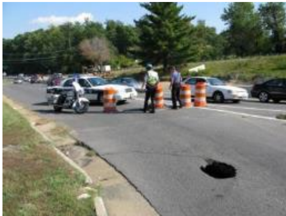
Sinks and their relation to solution cavities beneath the surface.
