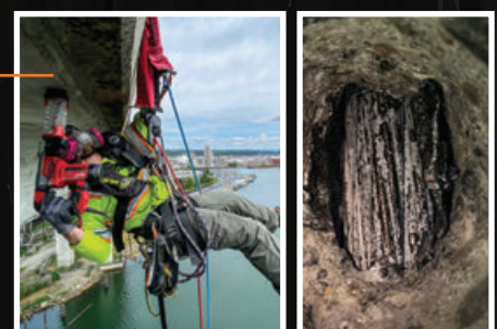
Physical sampling and borescope evaluation
